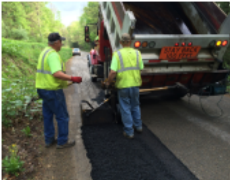
Road edge repairs with Moon Paver
