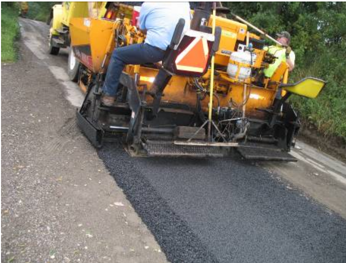
Laying down near the top
