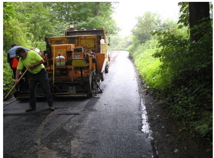
Starting second side, uphill
