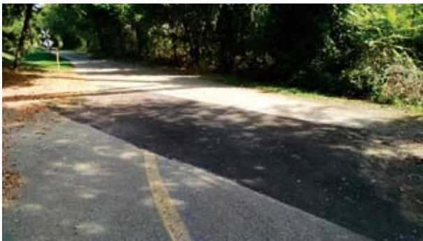
Schuylkill River Trail Repair
