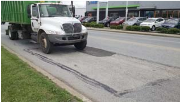
Ridge Pike Repair in Conshohocken, PA
