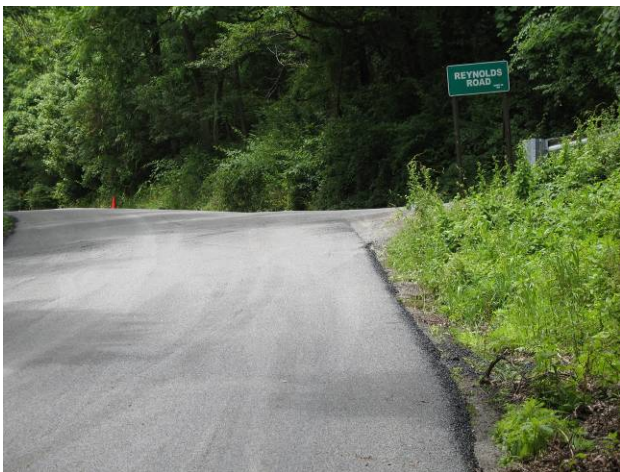
View uphill by Reynolds Road
